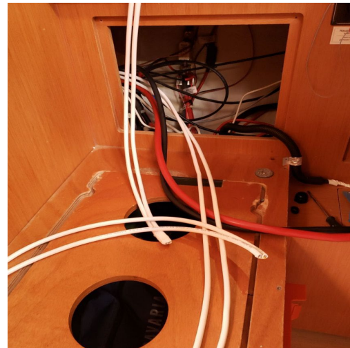
Fig. 16.12: Impressions of the cabling work.
