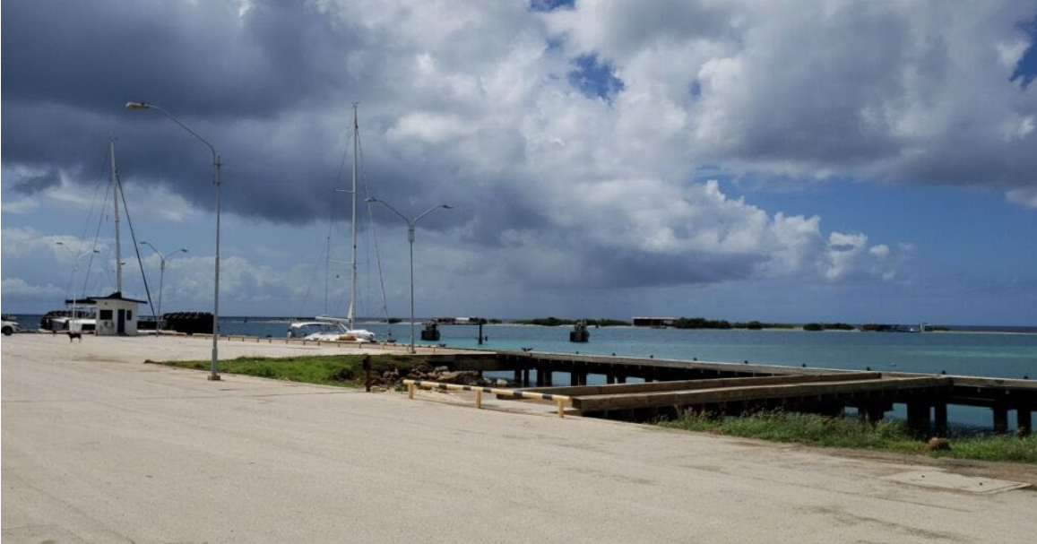
Fig. 33.22: The infamous wooden bridge. Tanuki is further ahead.
