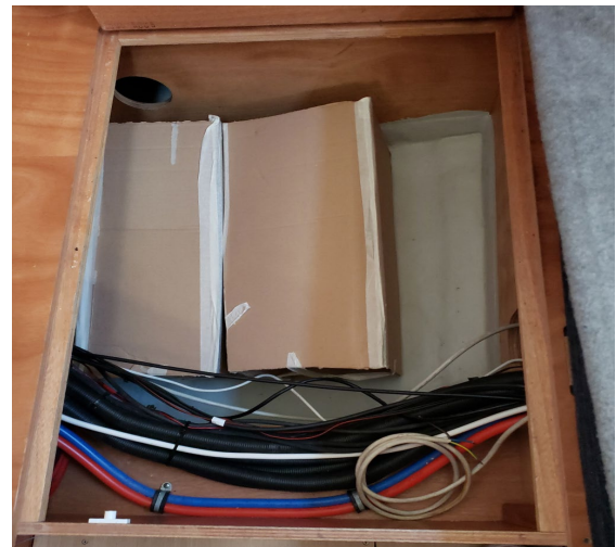
Fig. 8.9: This is where new batteries will go. Test fitting with cut-to-size cardboard boxes!
