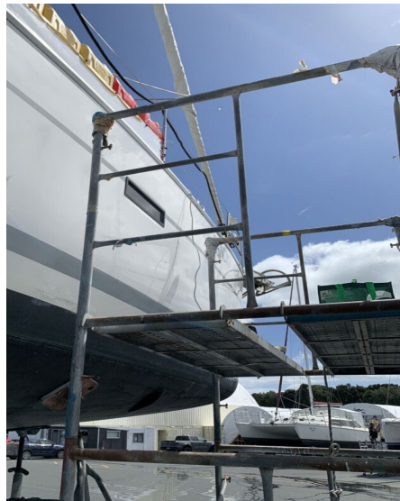
Fig. 54.29: Scaffold for polishing. Two days of work!
