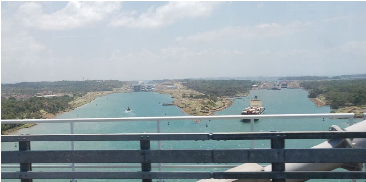
Fig. 36.1: The Gatun Locks as seen from the bridge. On the right, the traditional route; on the left, the new locks for the bigger "Panamax" ships.
