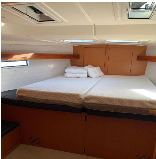
Fig. 7.11: The new owner's cabin after removal of the partition wall.
