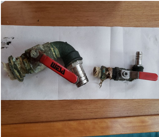
Fig. 26.15: The old seacocks removed.
