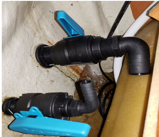
Fig. 26.16: New valves during fitting.
