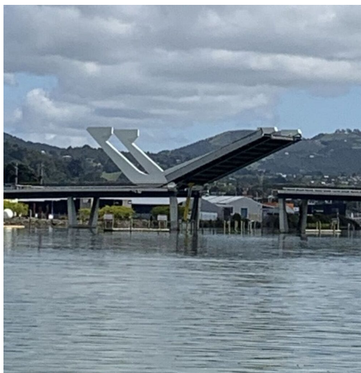
Fig. 54.4: The Hatea River bridge opens for us.
