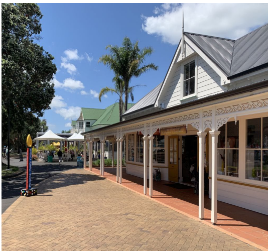
Fig. 54.8: Whangarei – Colonial-style houses.
