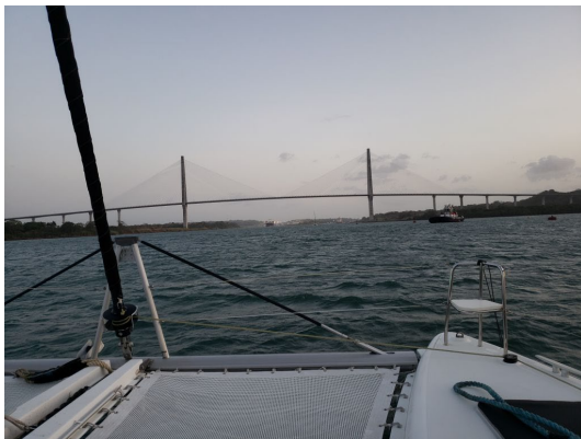
Fig. 36.2: Going under the bridge.
