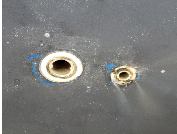
Fig. 26.14: Through-hull fittings from the outside. Already sanded down.
